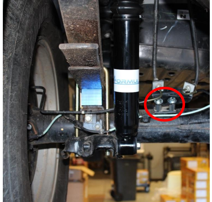
Picture 3: Installation of brake line spacer
